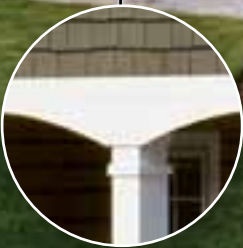
Restoration Millwork Wrapped Column and Routed Trimboard
